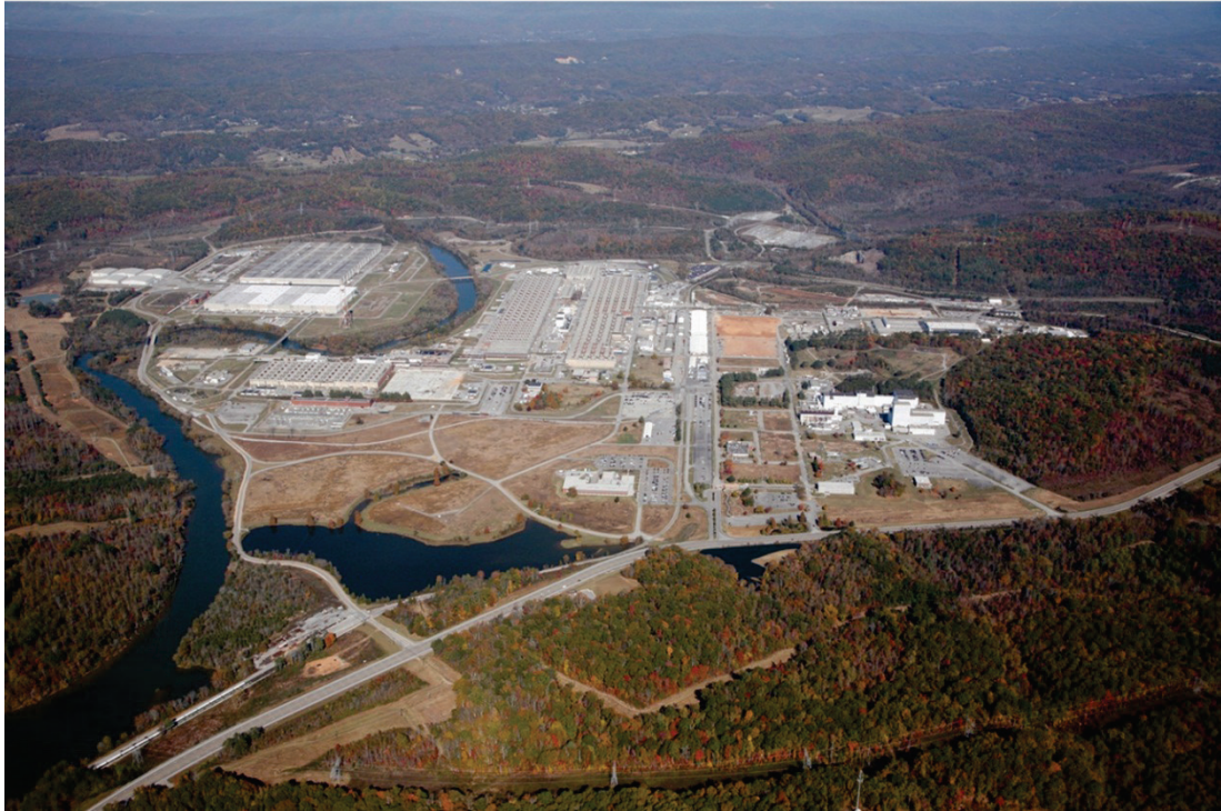
Fig. 3.1. East Tennessee Technology Park.
