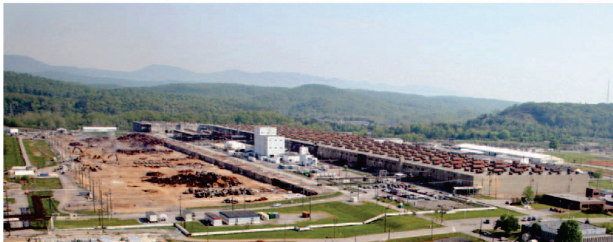
Fig. 3.63. Building K-25 after demolition of the west wing.
